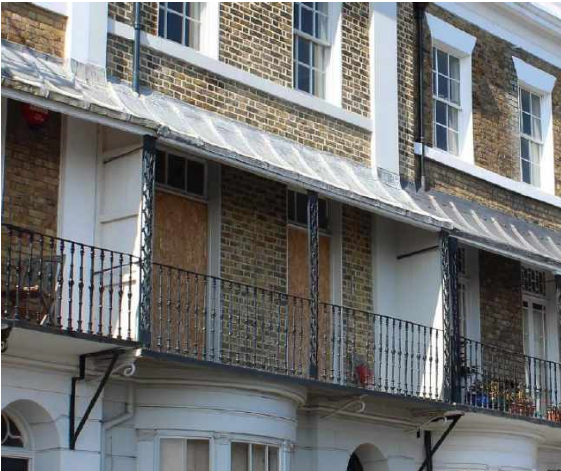
Iron verandah with lead roof, stucco details, brick in Flemish bond
